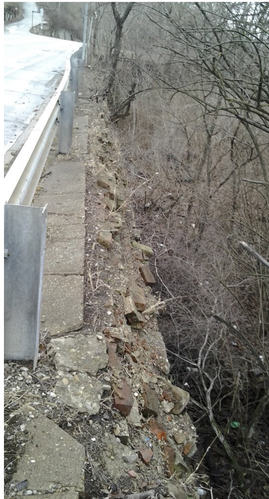
Riverside Drive Retaining Wall at Friendship Park
