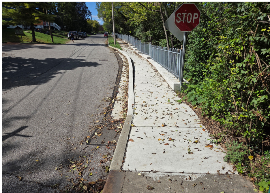
Maryland Avenue Wall Reconstruction Completed
