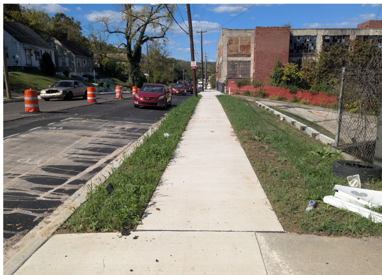
Beekman Street, Completed (Roadway Work Ongoing)
