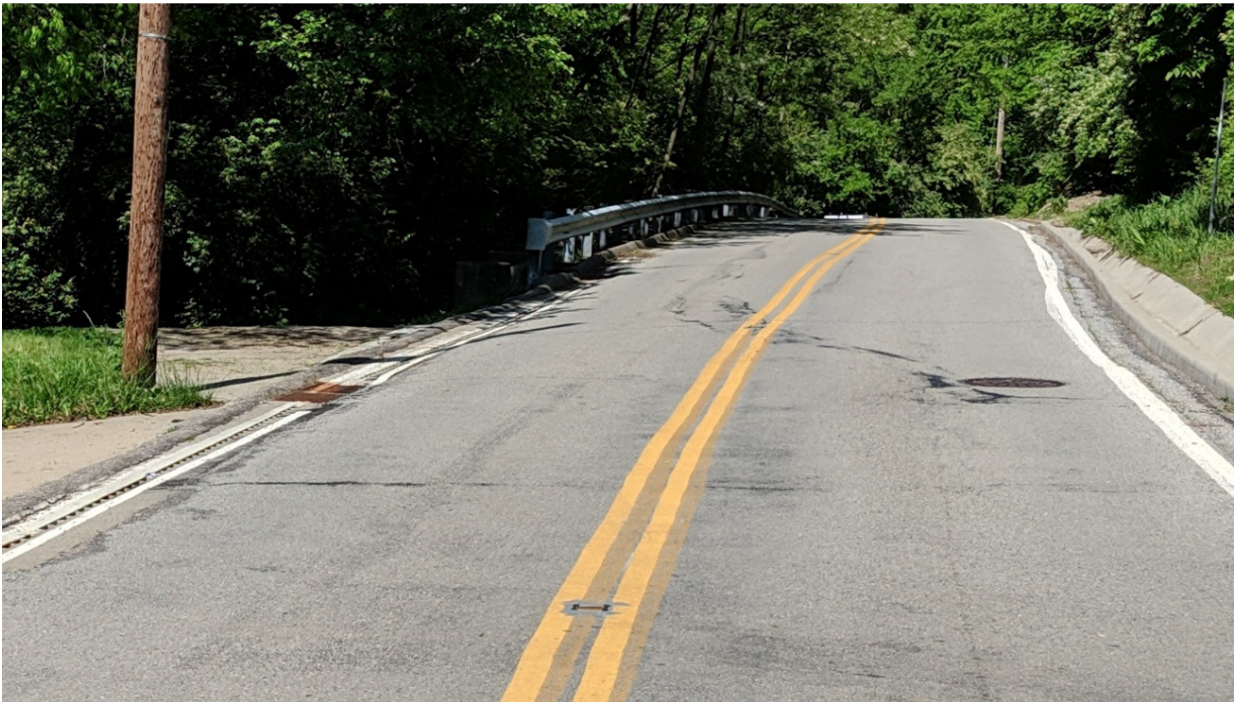
4291-4261 Hillside Avenue (Area 1)
