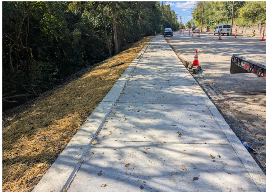
Harrison Avenue, Wall Complete, Roadway Work Ongoing
