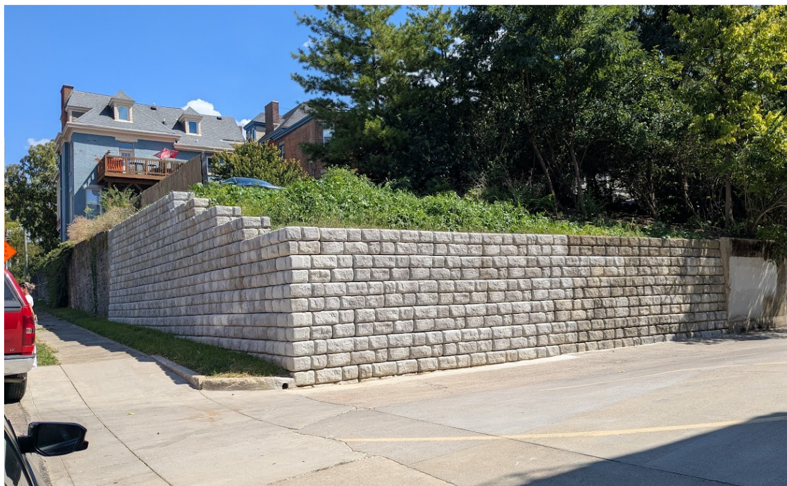
Eucledan Alley Wall Reconstruction - Completed
