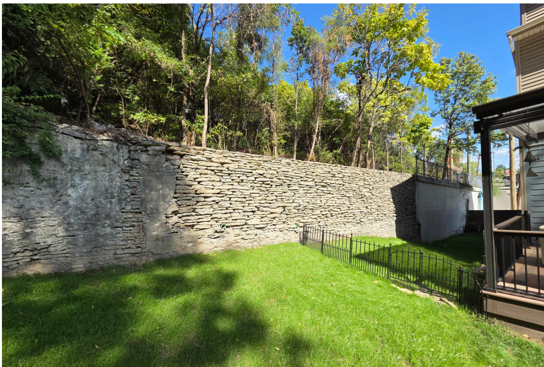
Sycamore Street Wall Reconstruction - Completed
