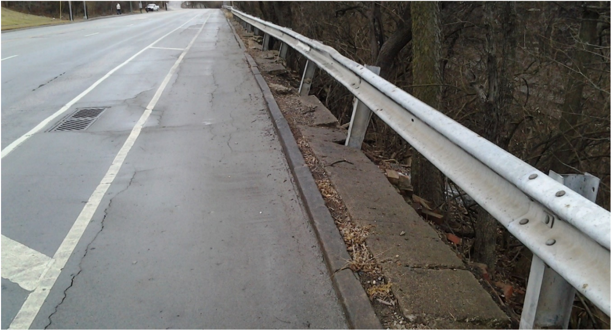
Riverside Drive Retaining Wall at Friendship Park
