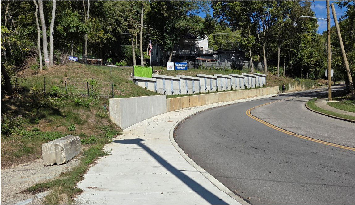
Anderson Ferry, Completed
