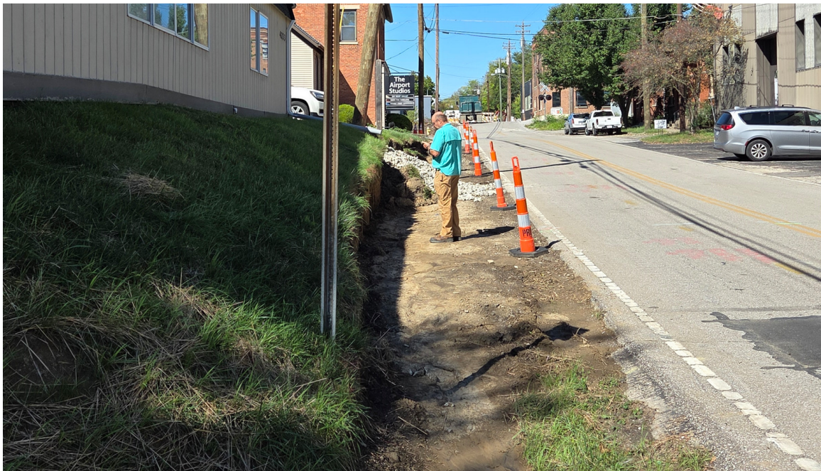
Airport Road Improvements – During Construction
