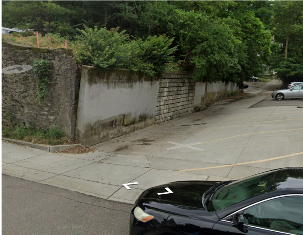
Eucledan Alley Wall Reconstruction – Before
