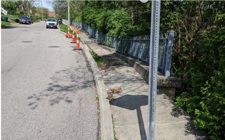
Maryland Avenue Wall Reconstruction – Before
