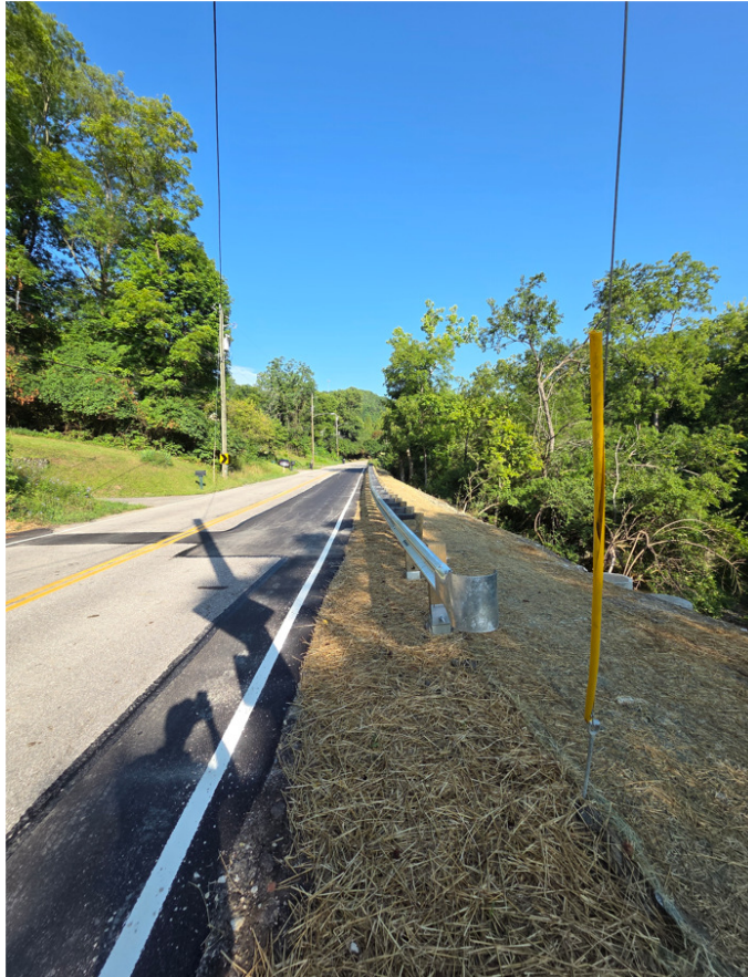
West Fork Road Landslide Correction, Completed
