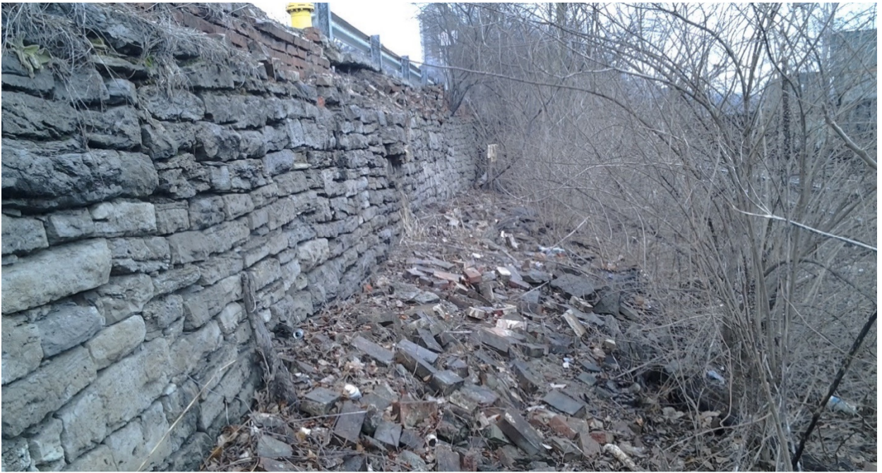
Riverside Drive Retaining Wall at Friendship Park
