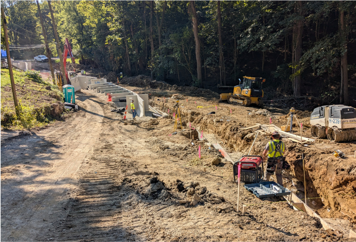
Yoast Avenue Reconstruction – During Construction
