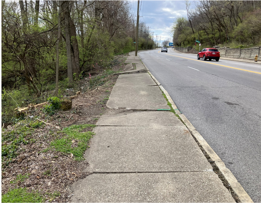
Harrison Avenue, Before
