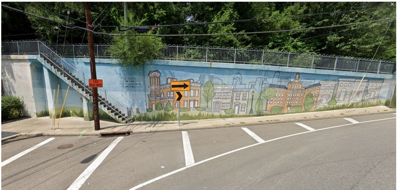
Sycamore Street Retaining Wall
