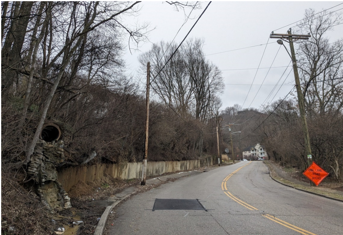
Anderson Ferry Road, Before
